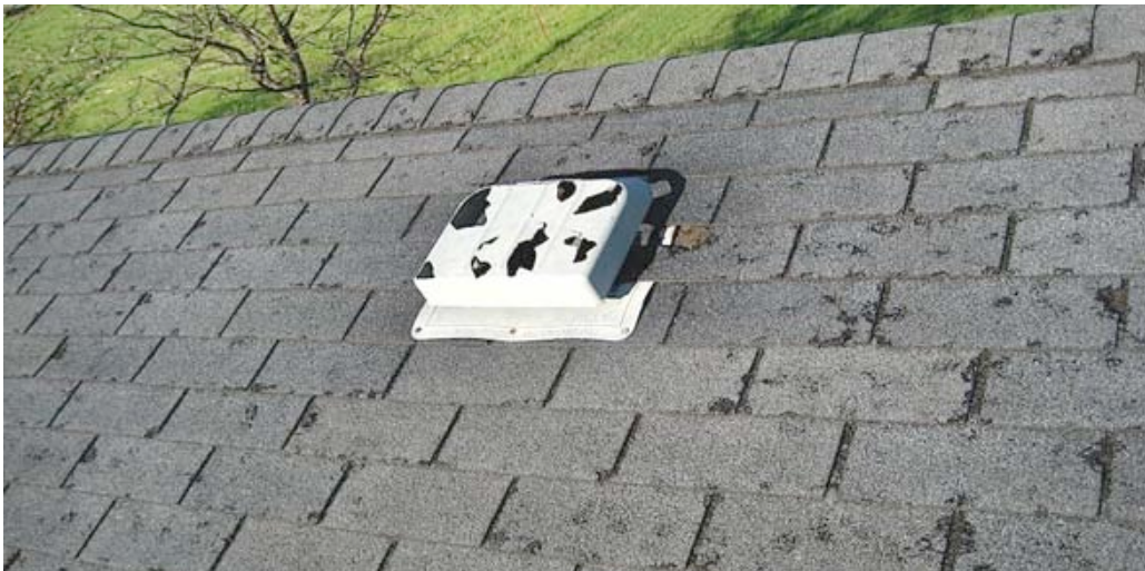
HAIL RIDDLED ASPHALT ROOFING DAMAGE- What The Professional Roofer Sees (While this picture shows substantial roofing damage hail “hits” are rarely ever visible from the ground & a responsible inspection means a professional getting up ON the roof)
